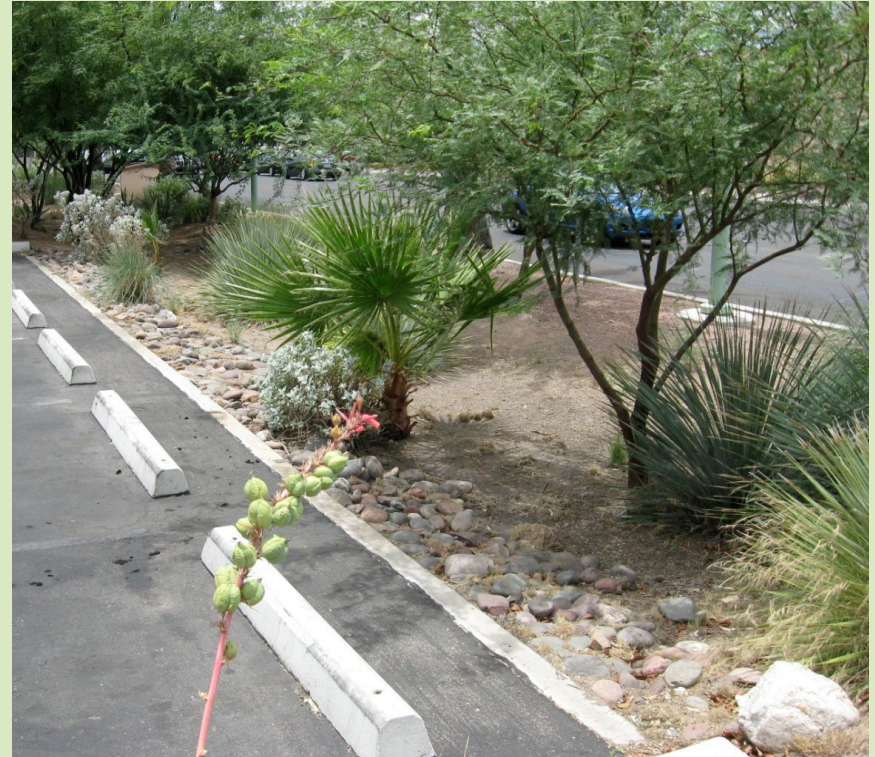
Parking lot designed to infiltrate runoff in Tuscon, AZ Photo Credit: Watershed Management Group
